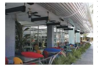
The Sunpak® Models S25 & S34 are outdoor rated heaters available for use with natural or propane gas. These heaters can be either wall or ceiling mounted. The optional mounting kit allows this heater to be mounted from above keeping the patio deck free and clear. Heat coverage varies depending on the wind exposure on patio. The average spacing between the heaters is 10 feet apart.
